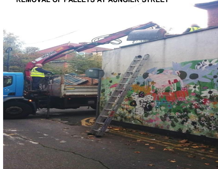
REMOVAL OF PALLETS AT AUNGIER STREET
